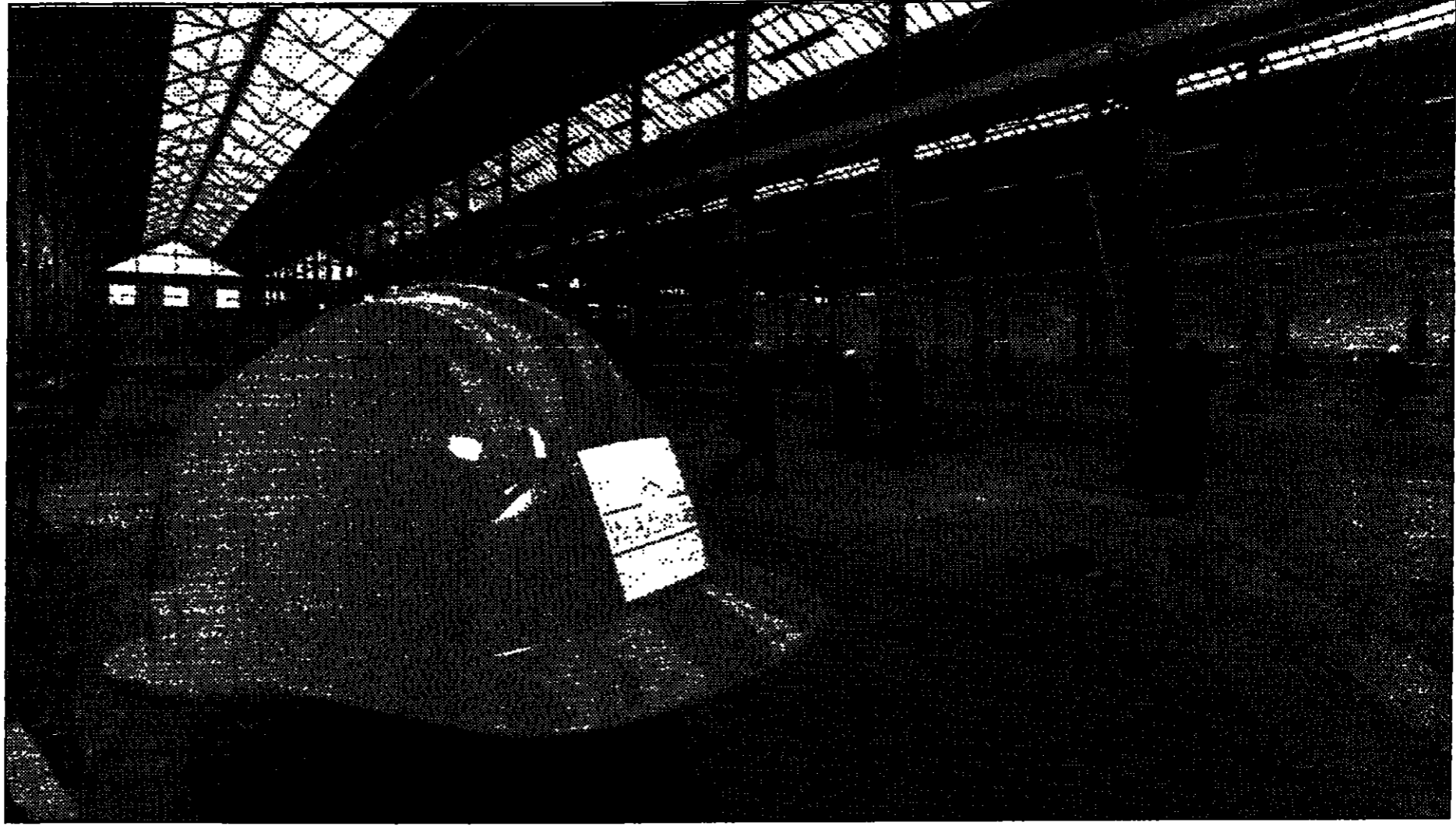
Heritage industry... Builders converting the Swindon foundry and boiler shop of Brunel's era into a designer mall. Below, how the food court might look PHOTOGRAPH BY GRAHAM TURNER
